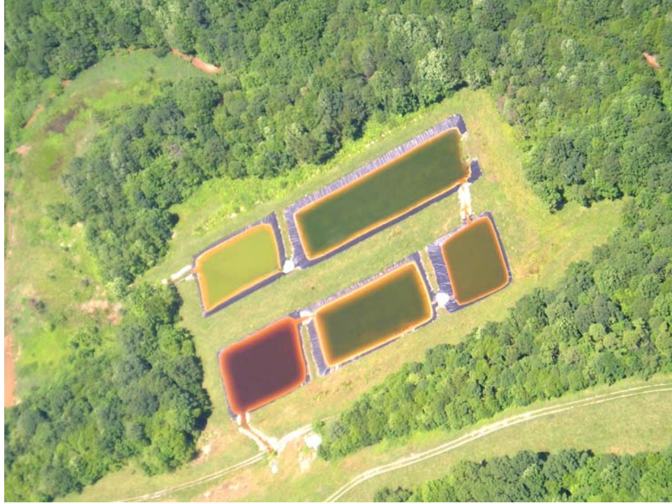
Photo 14: Reducing and alkalinity producing system installed near Kanesh Creek. The lower left pool contains a compost layer covering limestone, and the other basins are settling ponds.
