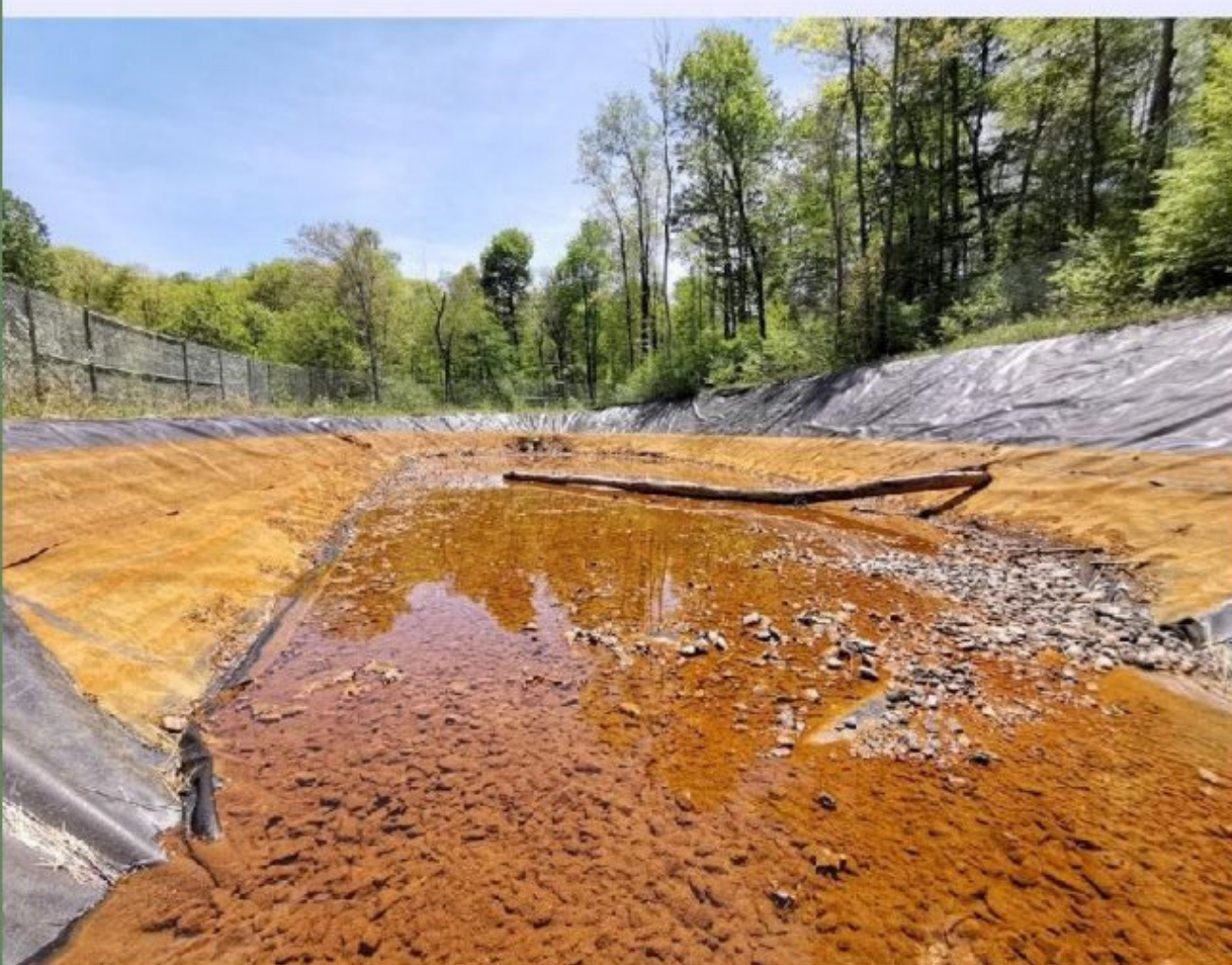
Ground-level view of the Satcher Pretreatment Portal
