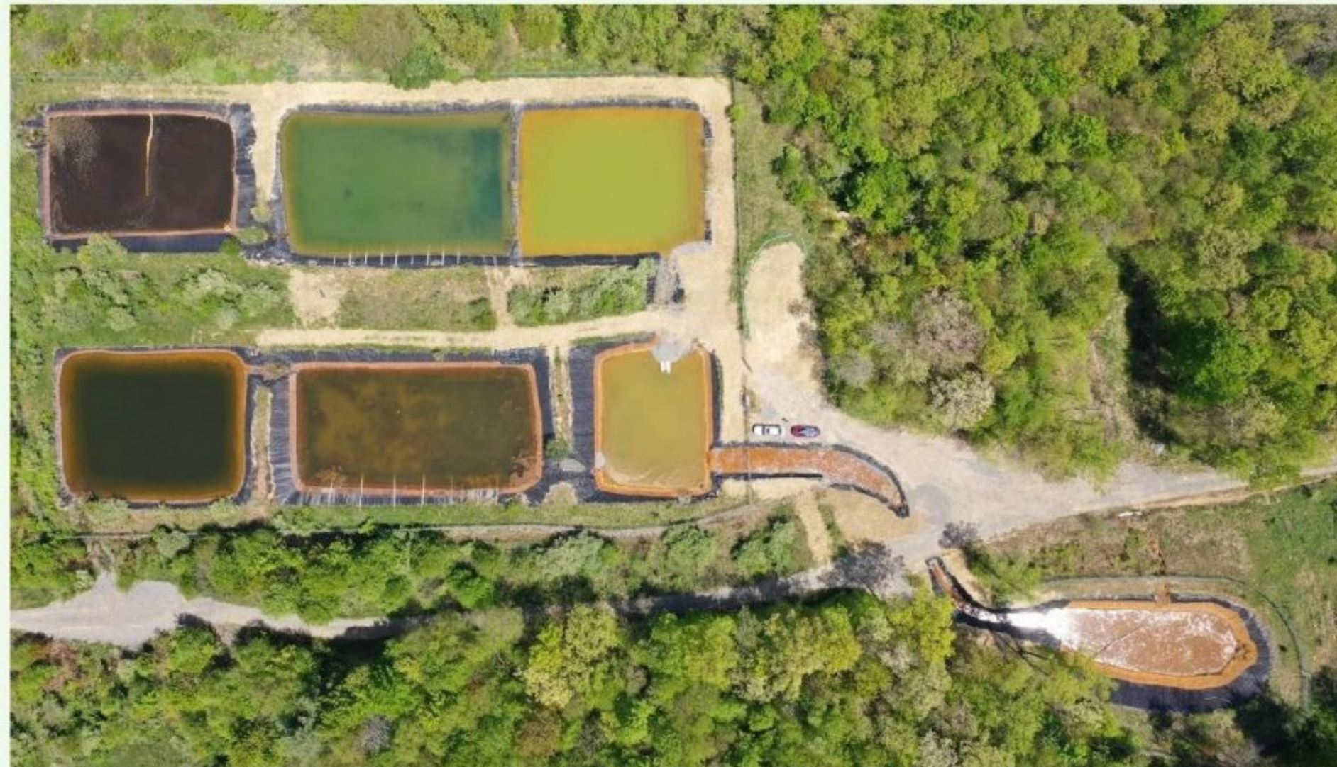
Aerial view of recently renovated Sandy Run treatment site.
