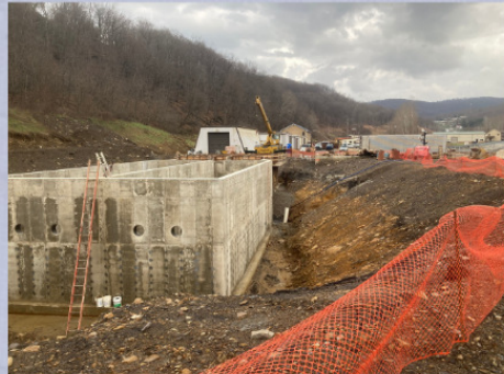
A look at the two clarifier tubs under construction.
