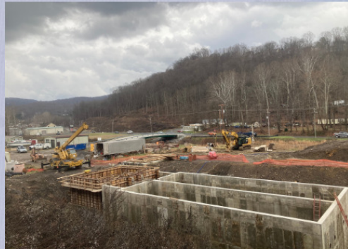
The Richard Mine construction site.
