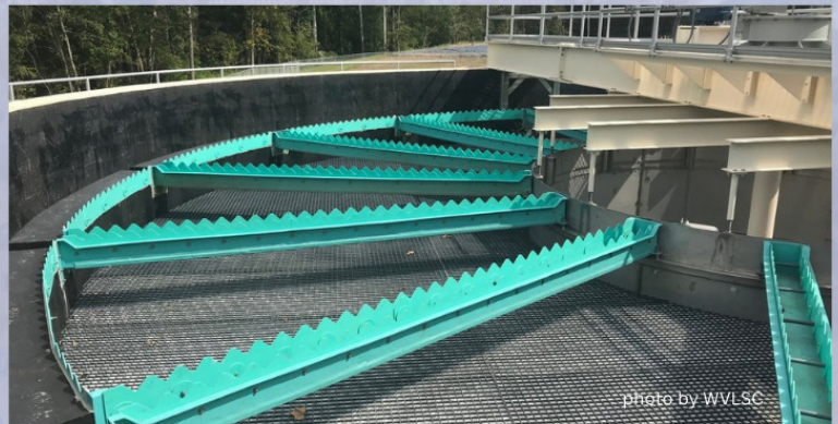
Clarifiers are part of modern acid mine drainage treatment.
