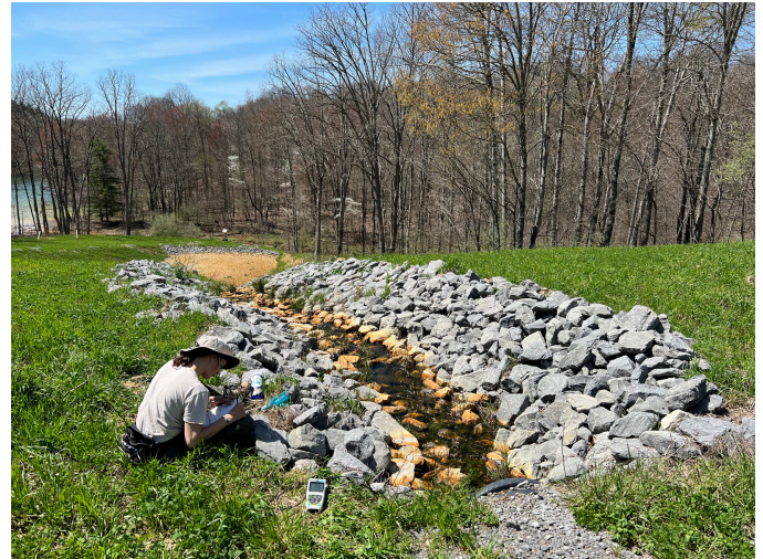
Photo: View from one of the open limestone channels.
